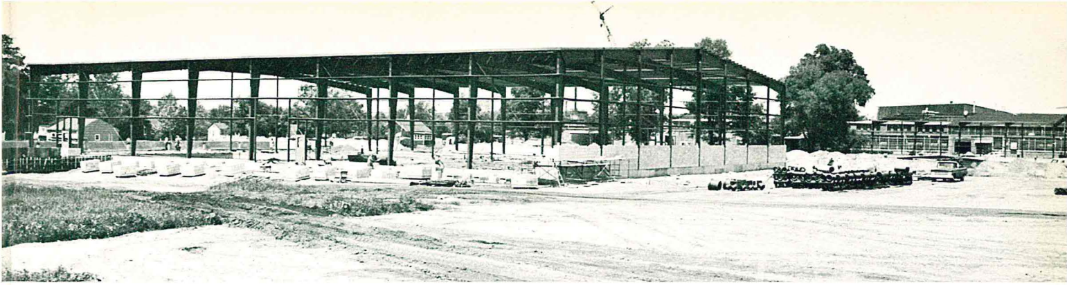
By the end of July the expansion program had progressed to this point—workmen were beginning to enclose the steel framework of the building which will house the research and development quarters and the customer demonstration areas.
